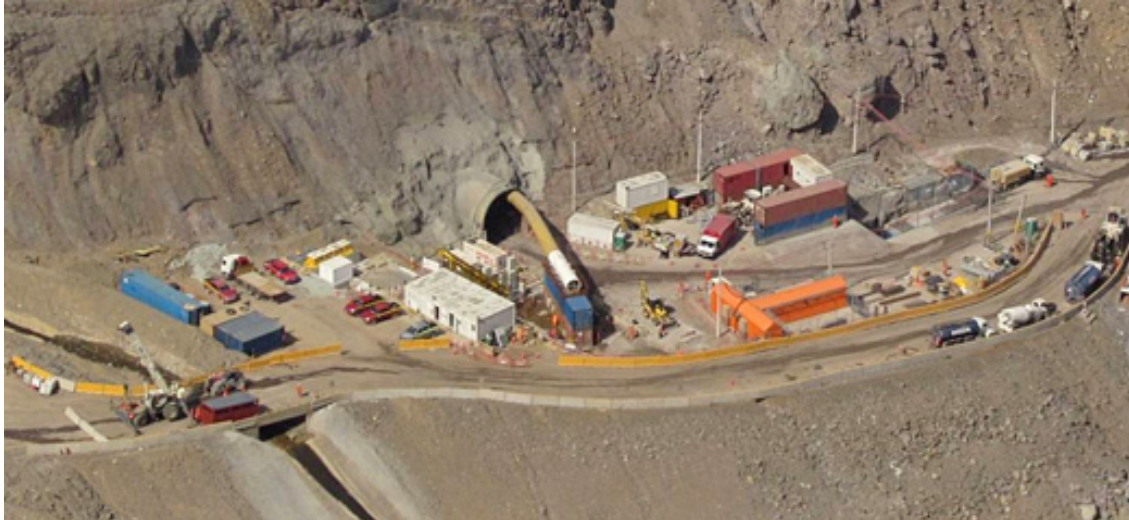
Figure A.7: Main entrance
